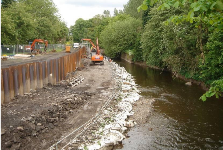
Photograph no 2 – Flood wall in construction in Cathcart
