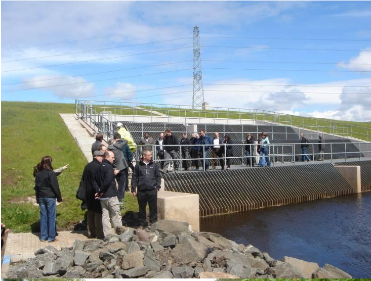
Photograph 1 – Inlet to flow control structure at Kirkland Bridge storage area
