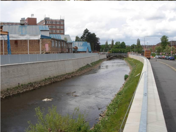
Photograph no 3 – Flood walls completed in Spean Street
