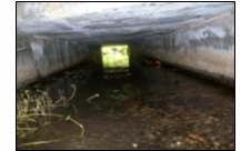
Ref 14 6/RN/As/SLB.50) Inlet of concrete box culvert at Drummond Road.
