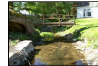
Ref 12 6/RN/As/SLB.46) Footbridge at 55 Drummond Road. Bridge size: 2.900x0.830 @ 900(wide)
