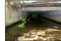
Ref 14 6/RN/As/SLB.50) Upstream of concrete box culvert at Drummond Road.
